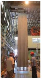
Finned water-cooled riser channels in the NSTF
