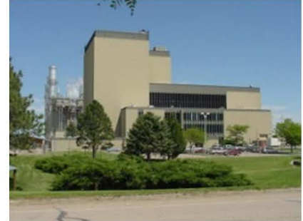
Fort St. Vrain (U.S.) 842 MWth prismatic ~800°C 1976–1989
