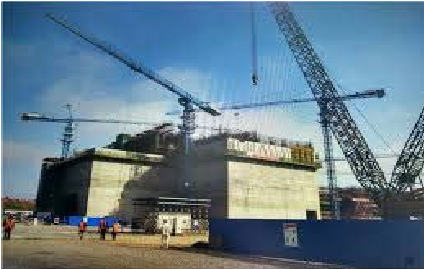
HTR-PM (China:2017-) ~2x100MWe Civil construction is complete
