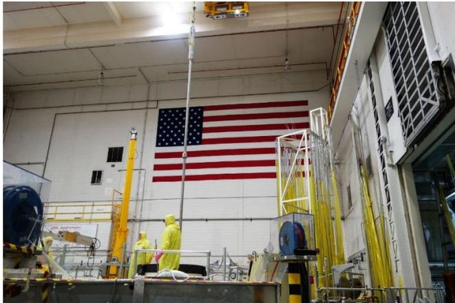
Test Train being installed in the ATR at INL.
