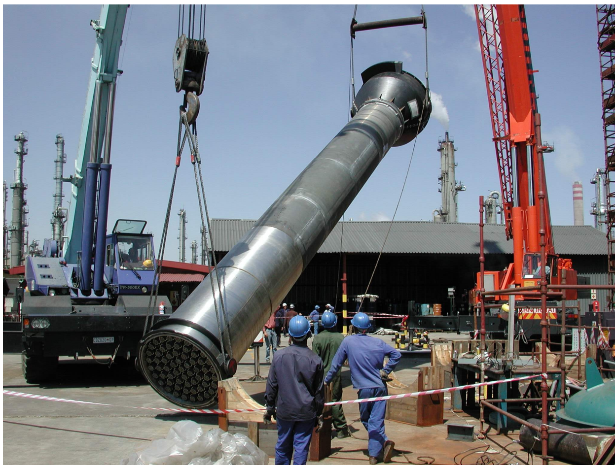
Figure G-2. Haldor Topsoe Exchange Reformer (HTER) internals being installed at Sasol facility.
