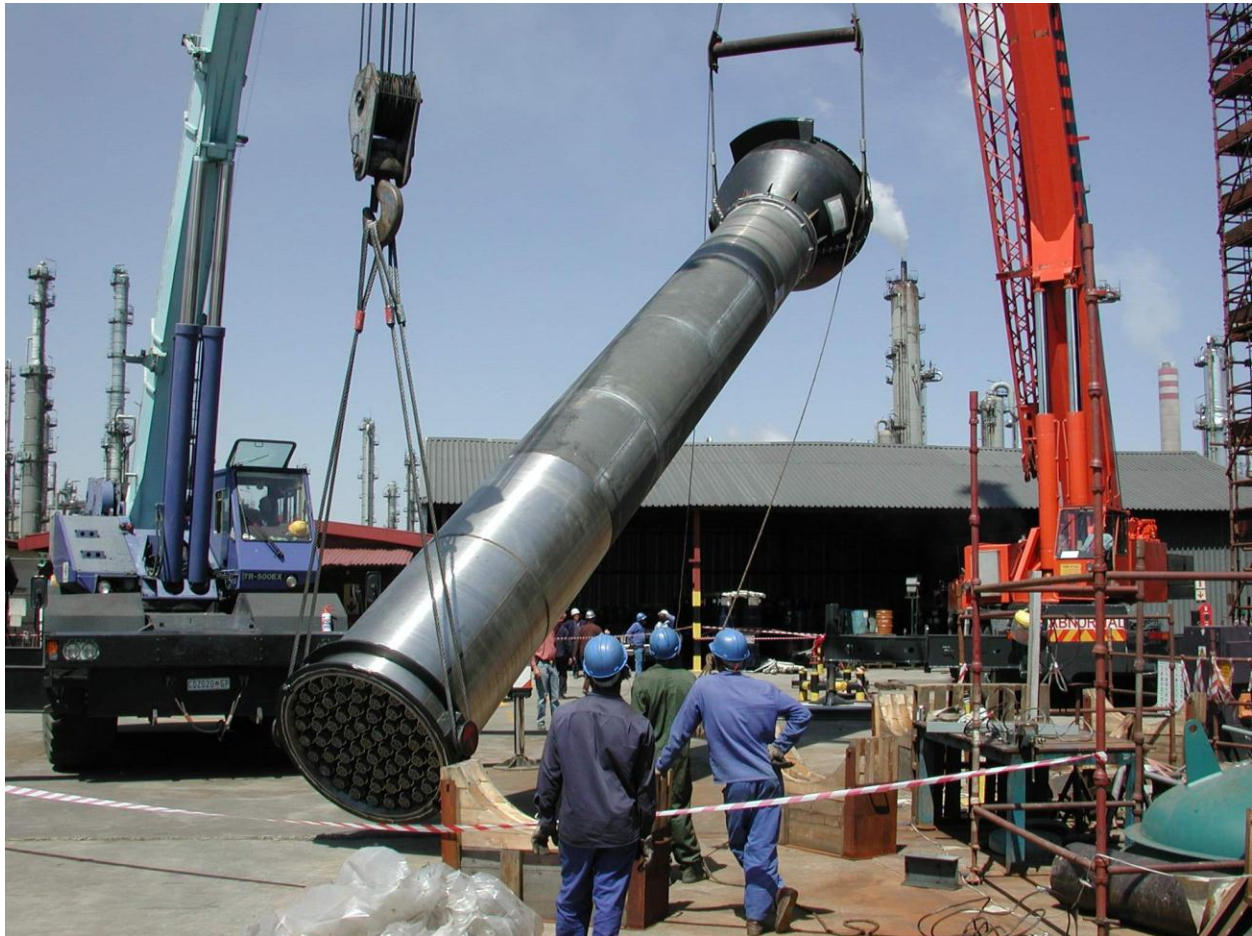
Figure G-2. HTER internals being installed at Sasol facility.
