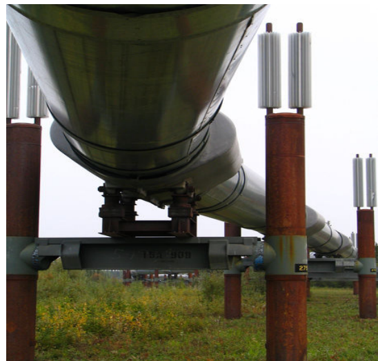
Figure 1-8. Typical vertical support member with heat pipes for trans-Alaska oil pipeline. b
