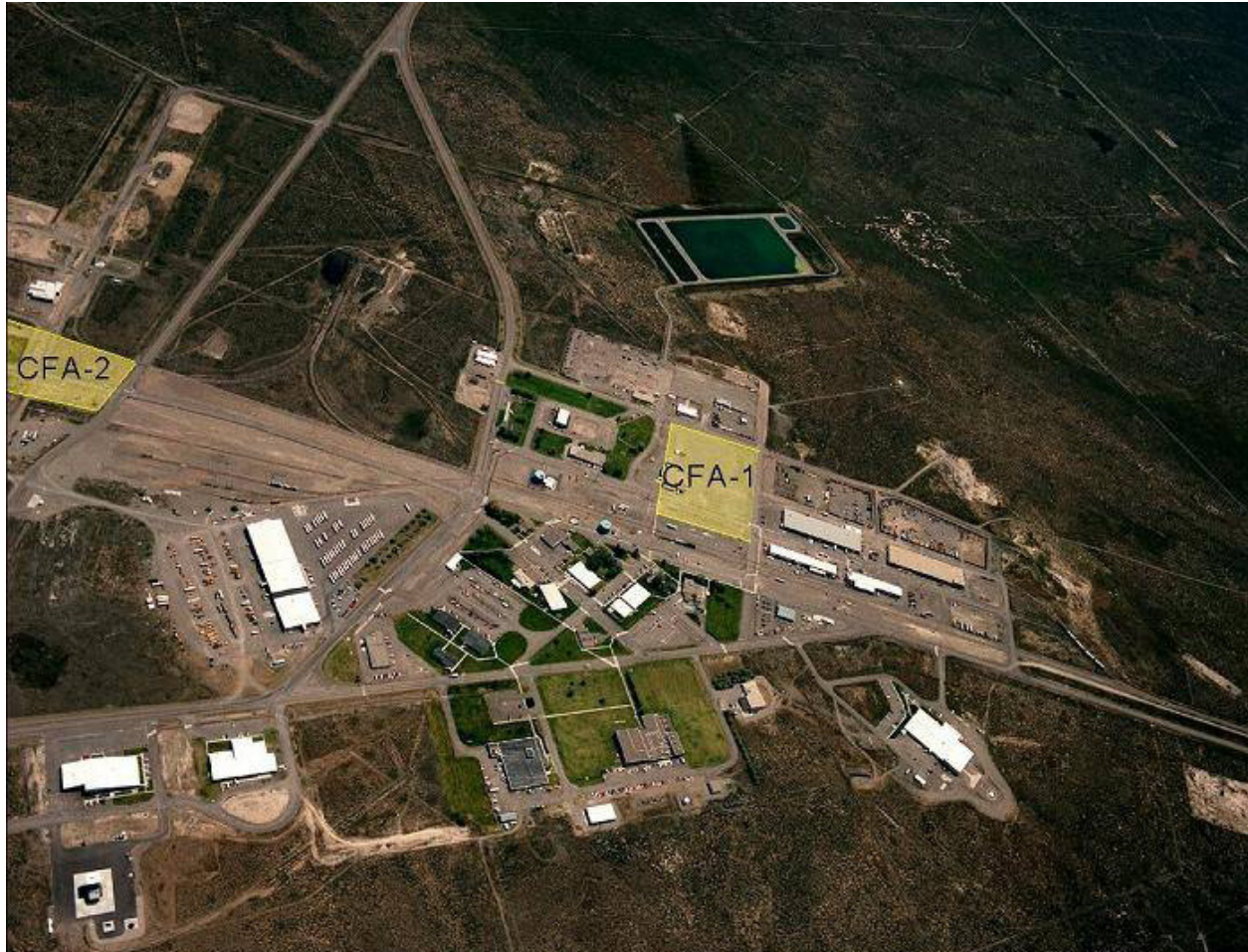
Figure 9. Central Facilities Area.
