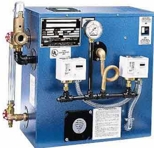
Figure 23. Sussman® low-capacity electric steam generator (27 lb/h, 0-90 psi steam).
